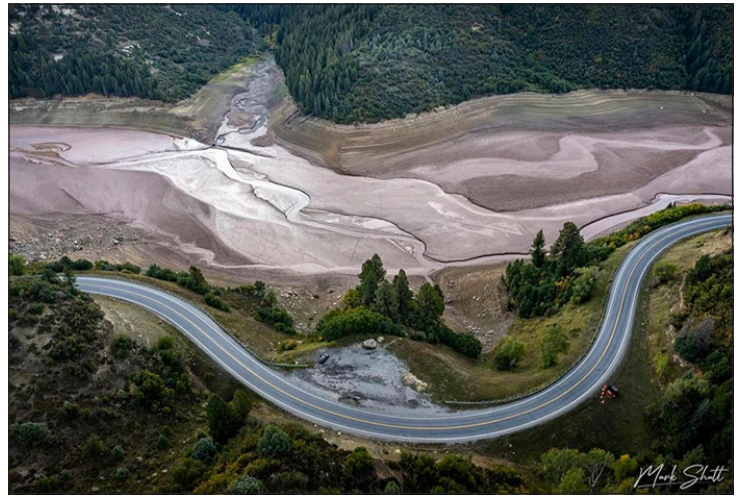
Paonia Reservoir, Colorado • Photo By Mark Shutt
