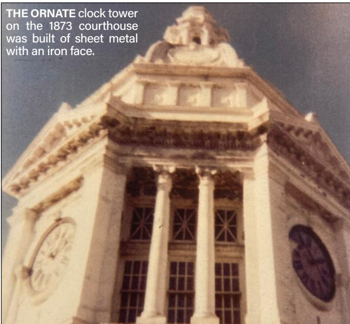
**THE ORNATE** clock tower on the 1873 courthouse was built of sheet metal with an iron face.
