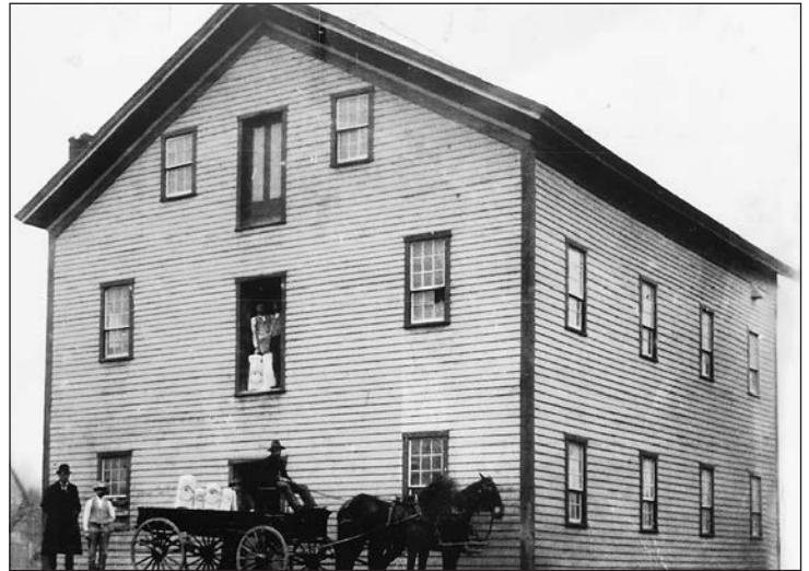
THE 1845 CHARLES MILL was a busy place in this late 1890s photo. Note the flour sacks. The building was later moved.
