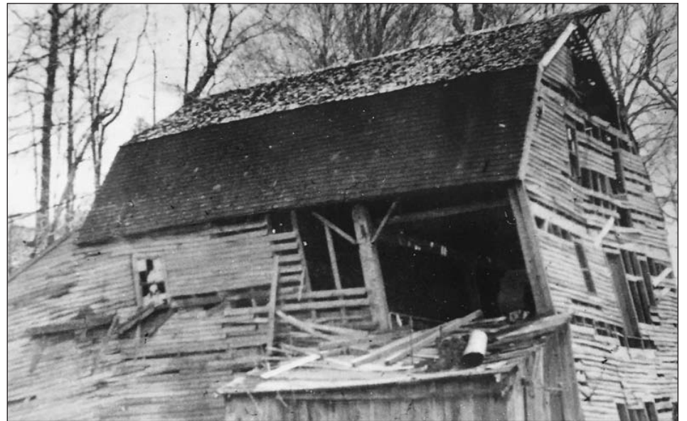
The last days of the old mill shortly before it collapsed.
