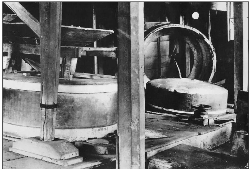
The interior of the Griebbling Mill shows one mill stone uncovered while the other has the hopper, hopper rest and hood still in place. The mill was leaning when the photo was taken.
