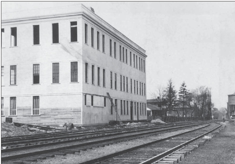
WORKERS put the finishing touches on the second Frye building after the first burned. It later became a basket manufacturer.
