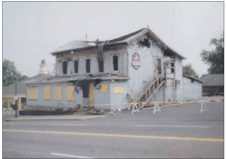
BUCKS was destroyed in a 1996 fire.
